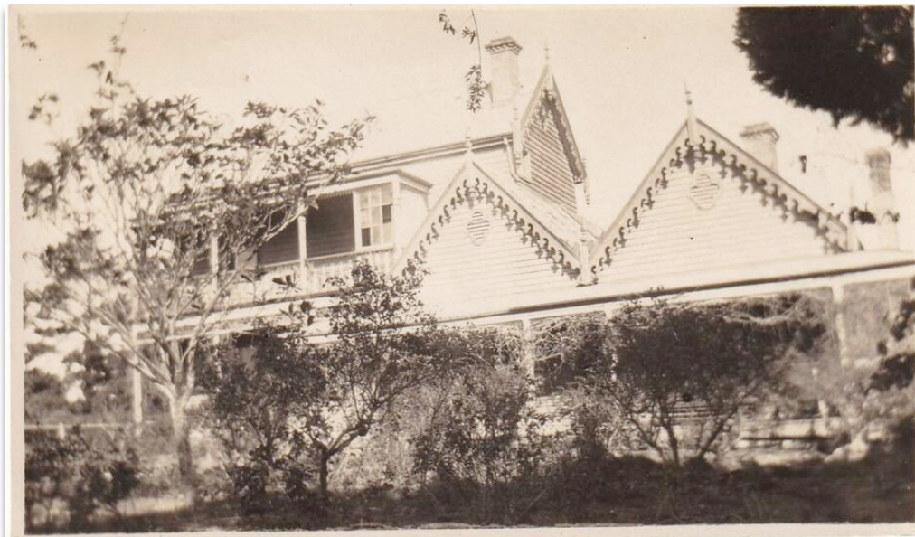
Image above clearly showing lacework and the turned timber finials and quatrefoil motif gable vents on Glen Isla.
