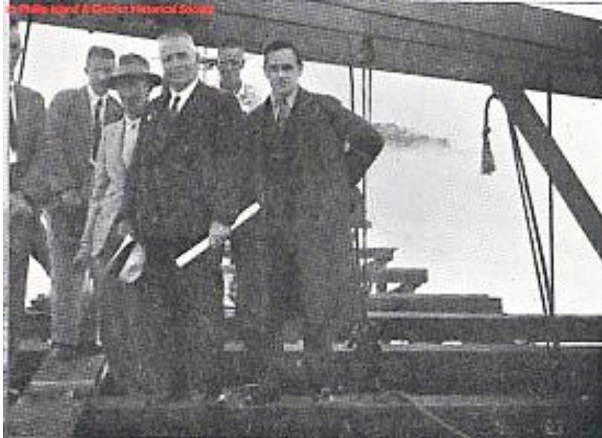
Group on first bridge under construction. Dick Grayden holding plans, Rupe Harris beside wearing hat. Phillip Island & District Historical Society collection.
