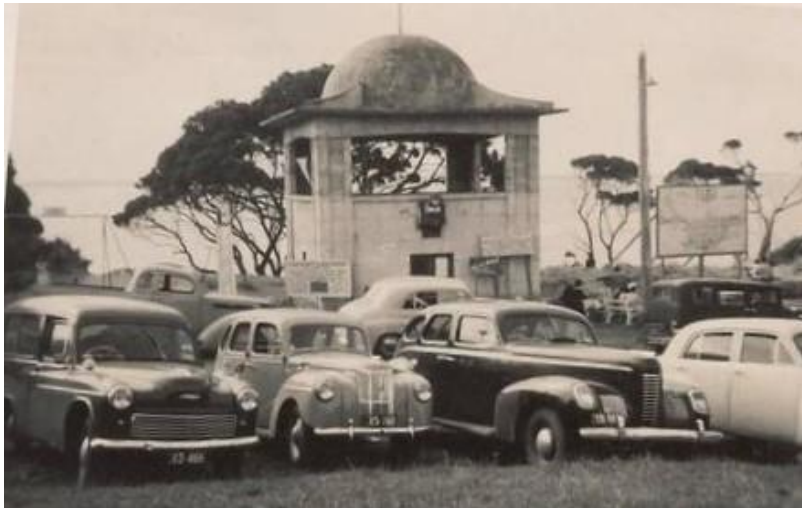
Band rotunda prior to upstairs windows being put in place
