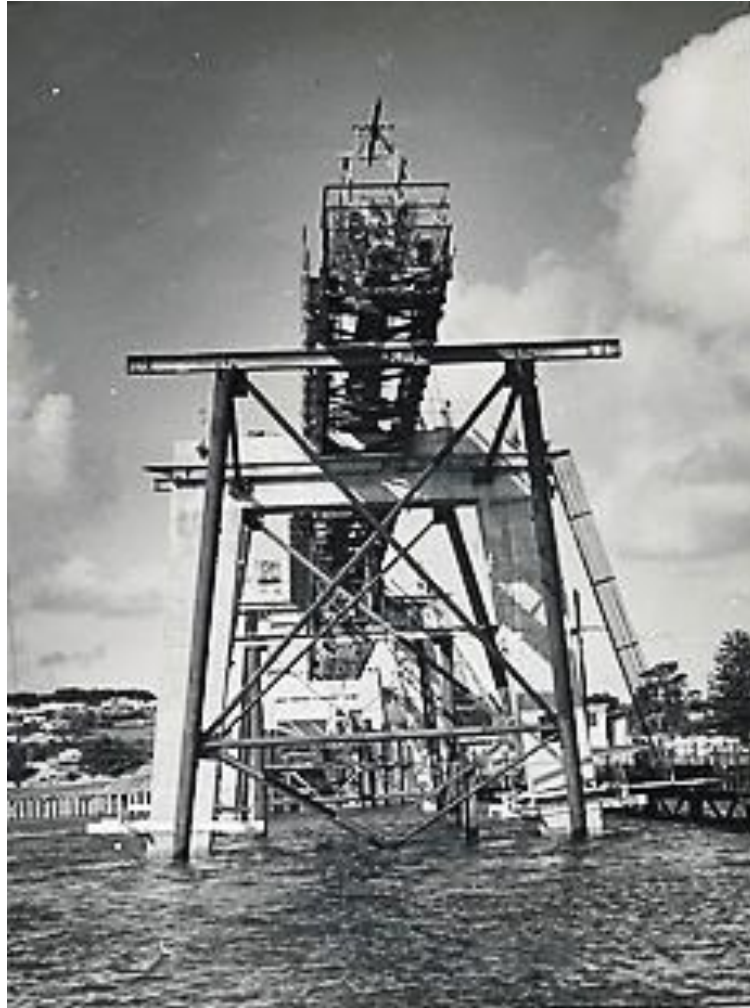
Second Phillip Island bridge under construction. Photo: Country Roads Board
