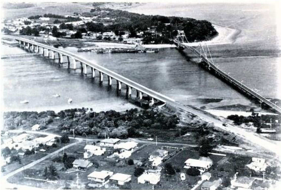
The two Phillip Island bridges before the suspension bridge was demolished.
